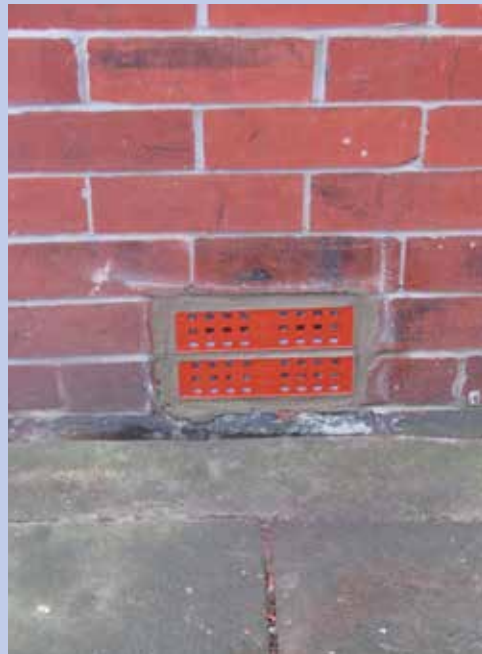
Image courtesy of Flood Divert
